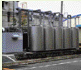
Soil Remediation Facility
