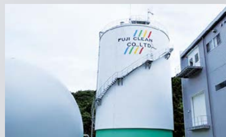
Exterior view of Fuji Clean Co., Ltd.'s methane fermentation facility
